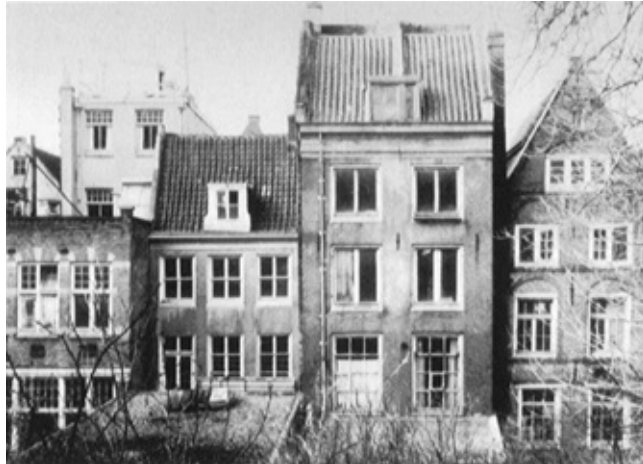
263 Prinsengracht, Amsterdam, rear view. The Secret Annex (top two floors and attic) as seen from the courtyard garden.
